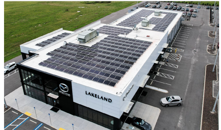
Mazda Lakeland's 412 solar panel installation.
